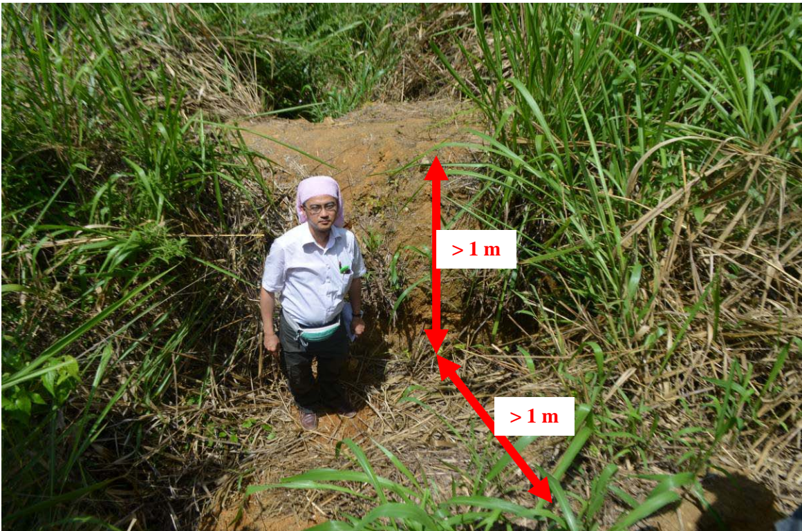
Figure 3: Large cracks and humps formed due to slope movement.
