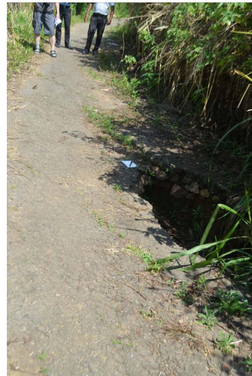
Figure 14: Damage to road along location GPS-2.
