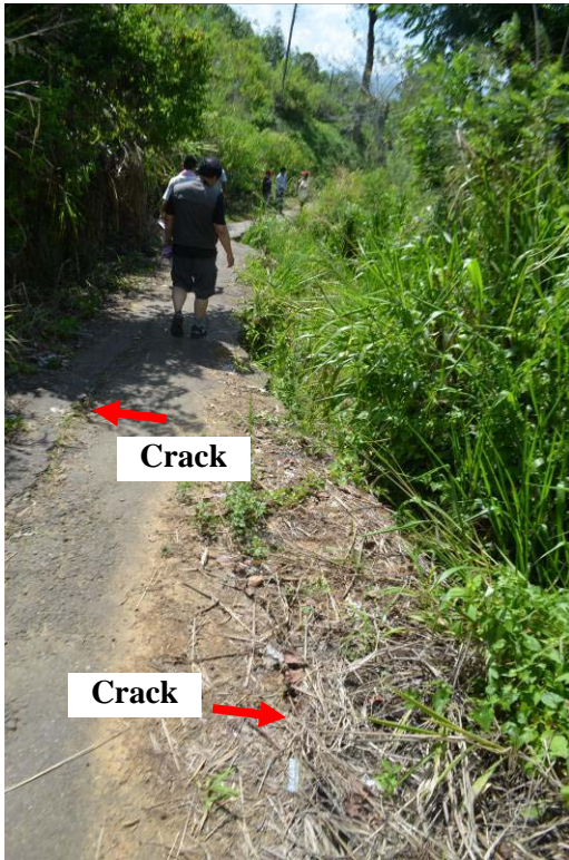
Figure 14: Damage to road along location GPS-2.
