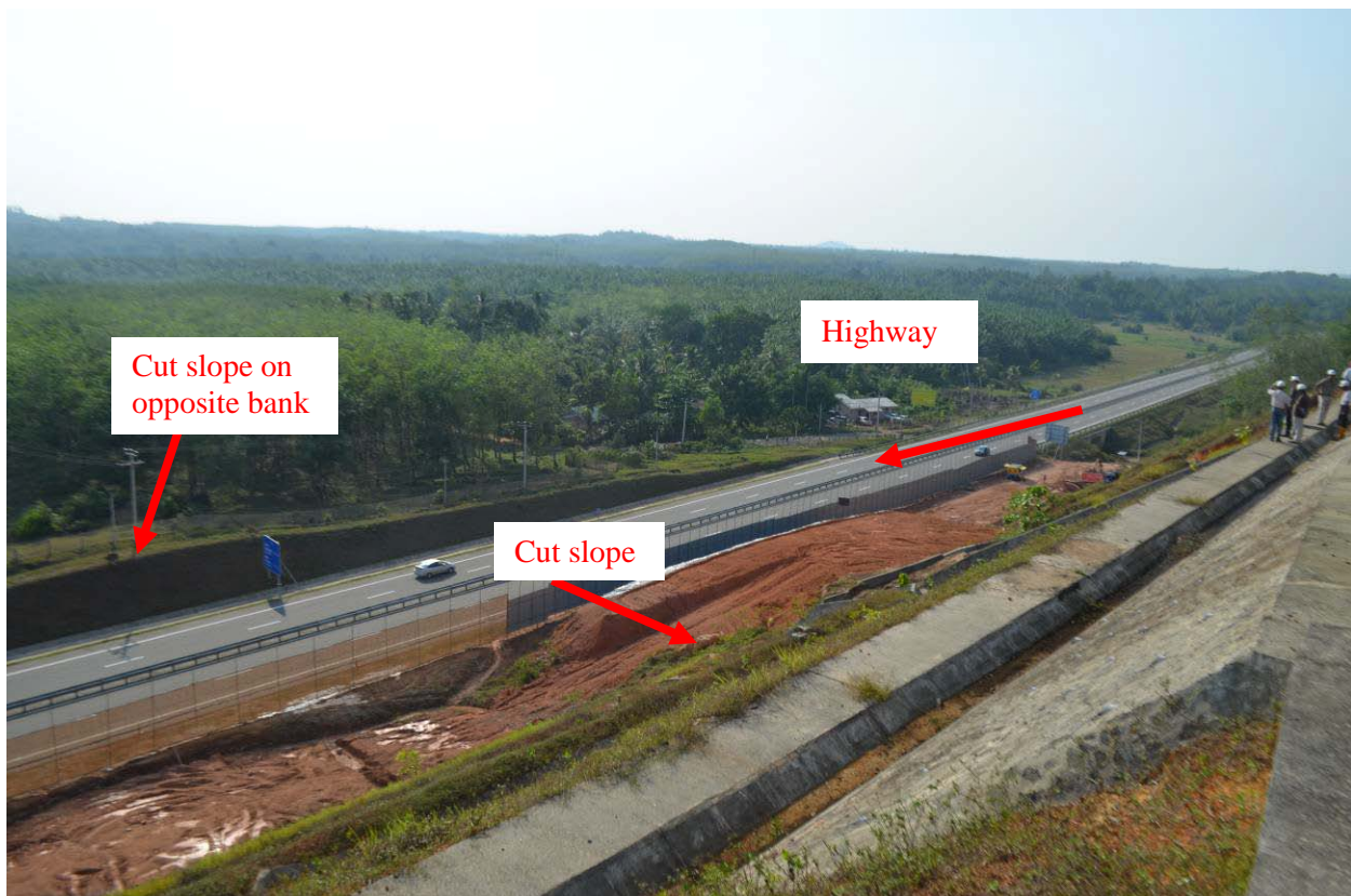
Figure 15: Cut slope to accommodate the highway
