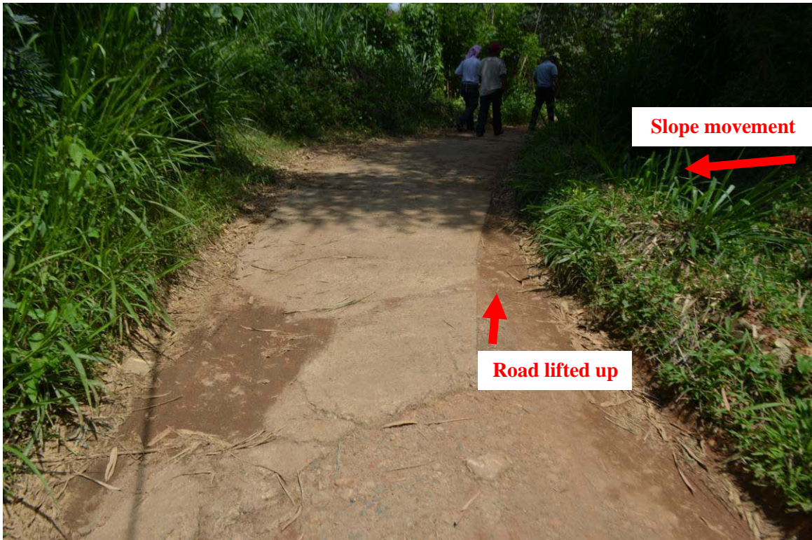
Figure 6: Deterioration of the road near the toe of slope.
