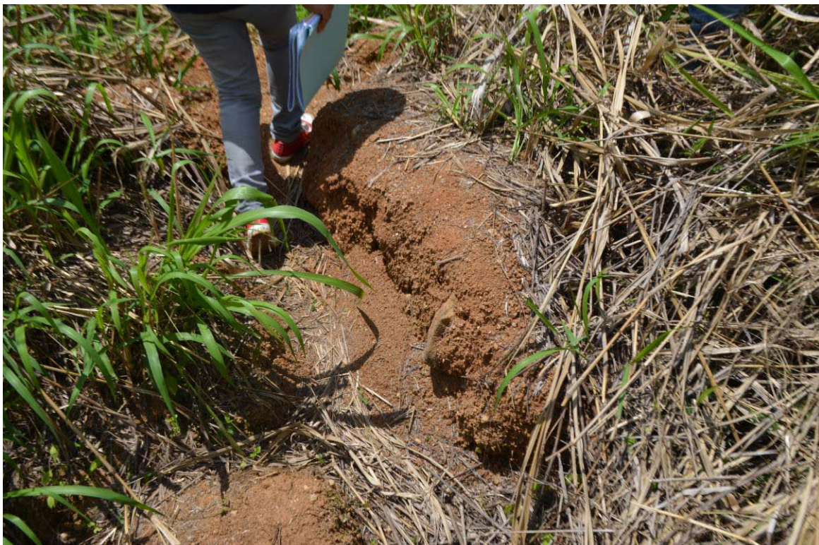
Figure 2: Visible cracks on slope surface.
